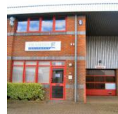
Framers Equipment Northampton
